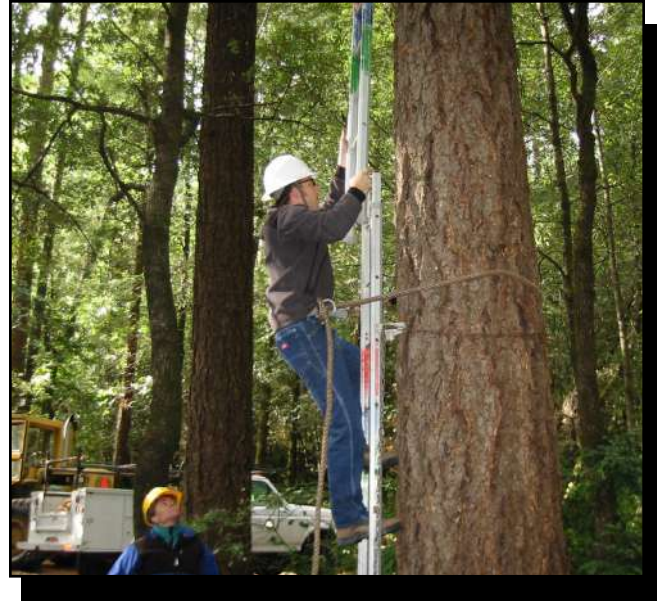
Figure 3—Increasing ladder heights by sections. The climber is secured to the tree by a climbing rope and the ladder is secured to the tree with a safety chain.
